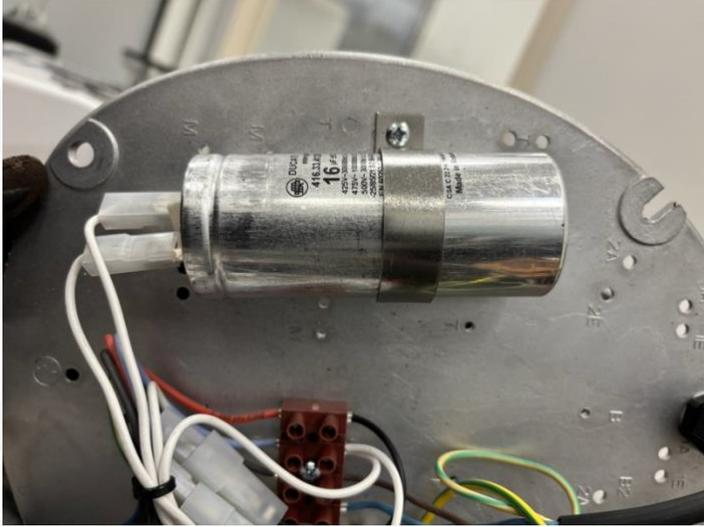
Remove the connections to free up the capacitor and remove the screws that holds the support //
